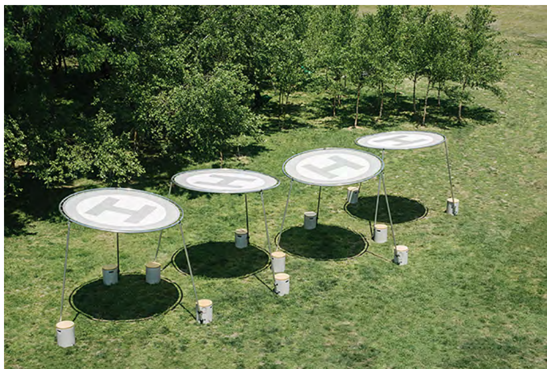
Circle Shade-2πR4 in a constellation of four units. Tilted shade canopies are lifted into the sky by a tripod pole structure anchored by cylindrical counterweights.
