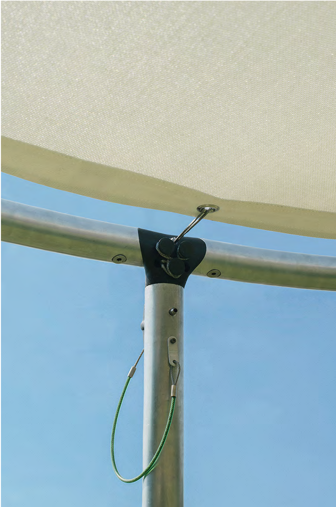
3D printed high strength structural node joint - cleats and embedded channel system integrate lacing of the canopy membrane
