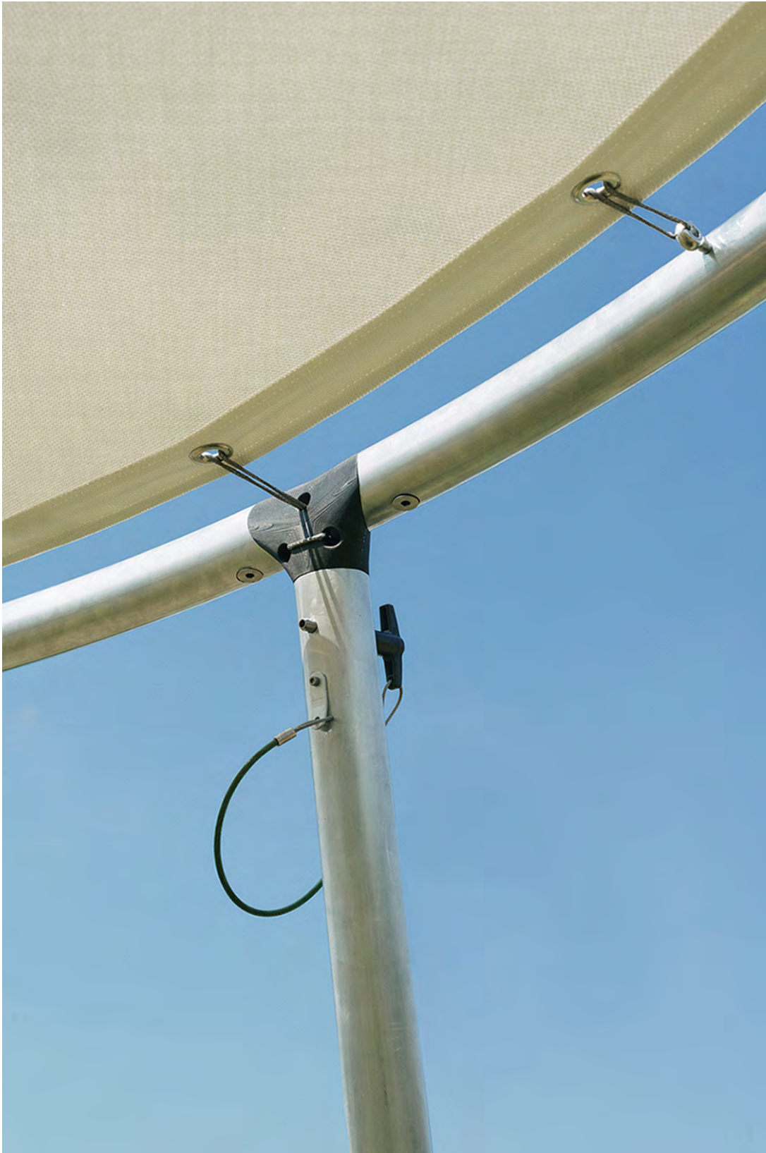
3D printed node with integrated channels for lacing of the canopy membrane
